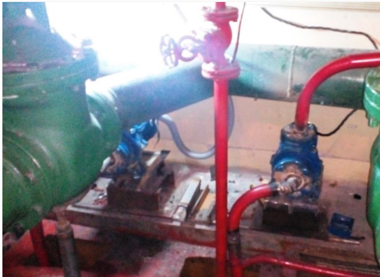
2 pumps, 45 m 3 /h each, instead of 10 m 3 /h for HEU zone
