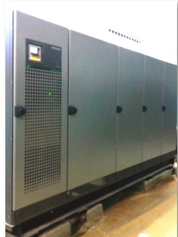
The batteries 30 kW, 6 hours
